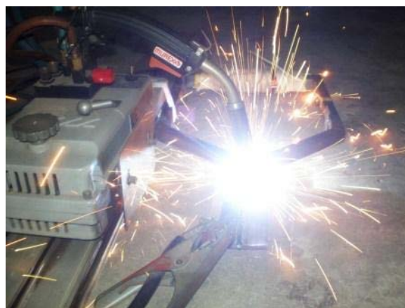
Fig 5. Automatic welding under external magnetic field.
